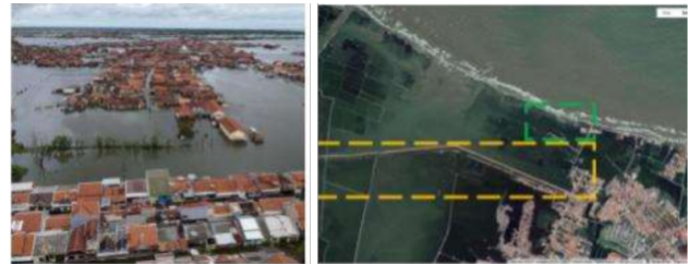
Fig. 2 Left: Flooding in Indonesia. Right: An existing sea wall (yellow) and mangrove grove (green) in Pekalongan. Figure adapted from [45]
